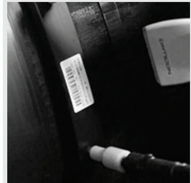
**3.** Scan the barcode with the barcode scanner and check that the weld time marked on the fitting is displayed on the control box display. For manual fittings, check the weld time marked on the fitting and enter this figure into the control box.
