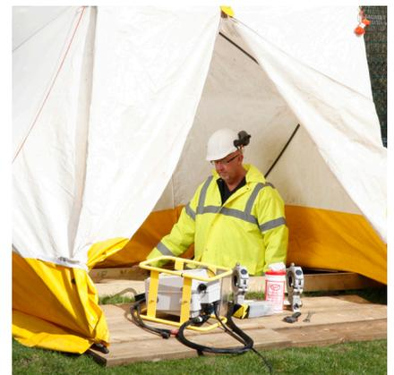
Ensure that the area where the weld is to be carried out has surface water removed and some form of groundsheet is used to isolate the jointing area from the trench floor.
