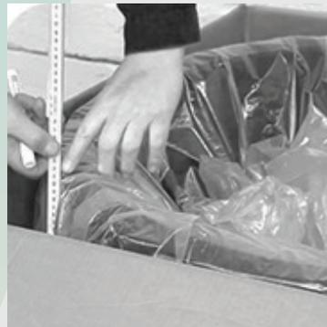
6. Cross hatch the area to be scraped plus an additional 20-50mm using the indelible marker pen.
