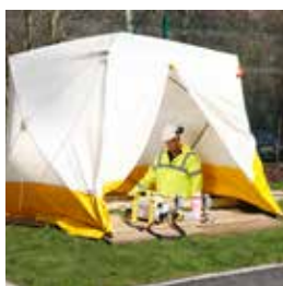
Welding tent/shelter and ground sheet
