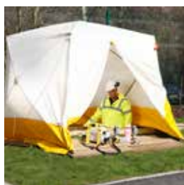
Welding tent/shelter and ground sheet
